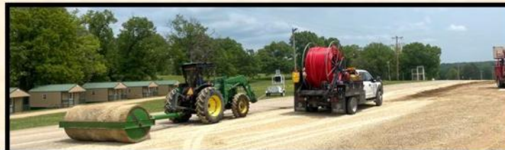
Gravel Added to Big Top Parking Area!
