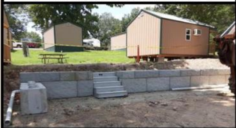
NEW STAIRS INSTALLED
